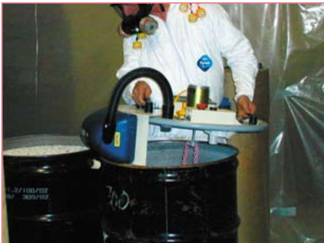
Источник: G. Helms (US EPA, Office of Solid Waste) Drum-Top Crushing of Mercury Lamps [ http://www.leirecycle.com/images/images_LRC/EPA_Drum_Top_Crusher_Powerpoint.pdf ].
